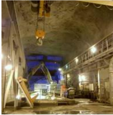
Palabora, storage hall (16x60x20m), Drakensberg (16x200x45m)
