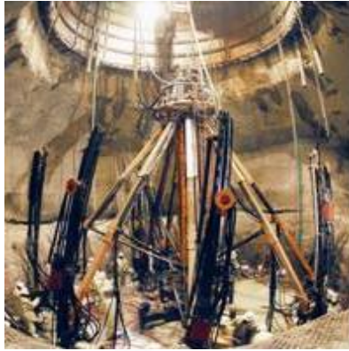
Impala 17, main shaft IPS station
