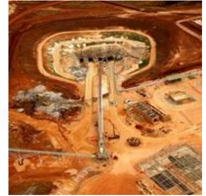
* Mining and Engineering Technical Services – full EPCM solutions
