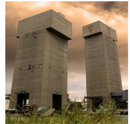
Palabora copper mine
