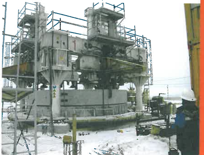
Early photo of the Russian contract showing a Herrenknecht shaft boring machine working on the presink of the 1 100 m deep shaft for client Eurochem. This photo also gives some idea of the weather conditions the Shaft Sinkers' team is having to contend with in winter (photo: Shaft Sinkers).
